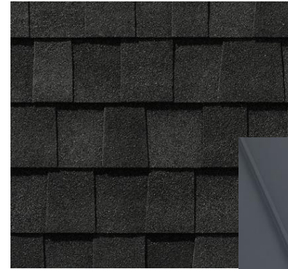
Asphalt Shingle Roof
